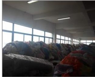
Photo of non-conformity Combustible materials such cloth production stored under the lights directly.jpg
